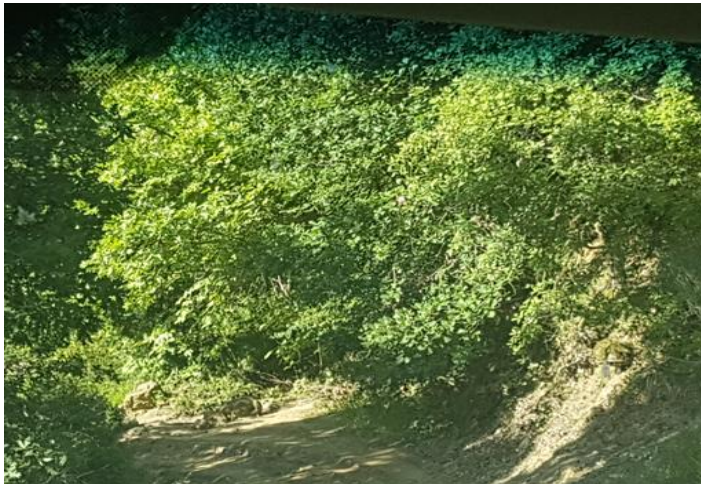
Figure 4-49: Example of unpaved, steep access road to village (Fratar village, Kelcyre Municipality)
